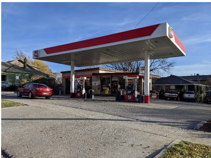
Figure 10 – Gas station and auto repair at 860 E 3 rd Avenue.
